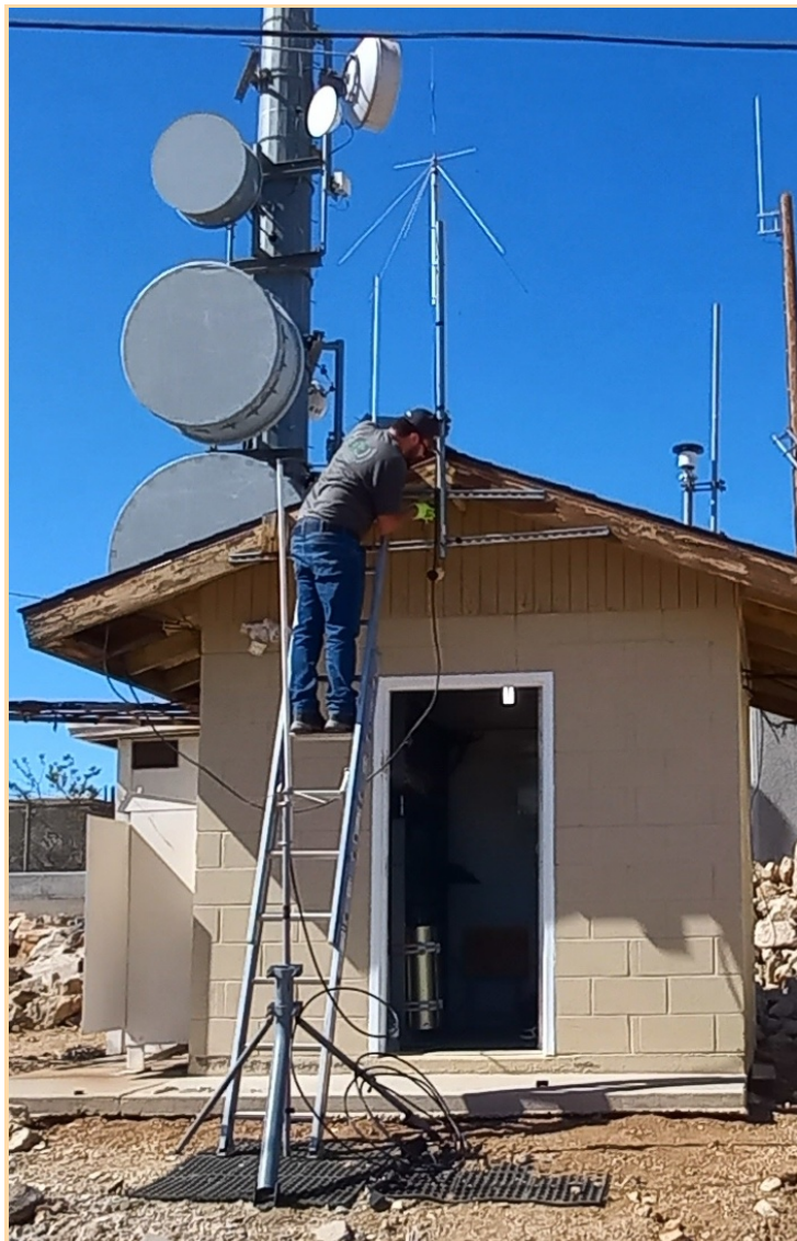
Byran KF6YGK mounts the discone antenna providing reception for the OpenWebRX+ SDRs. – Photo by KO6DAV
